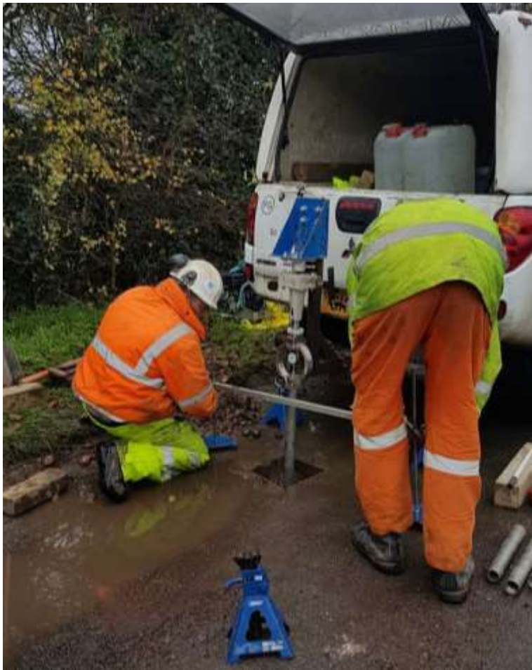
Figure 2.2: Operators carrying out the plunger penetration method at CBR01
